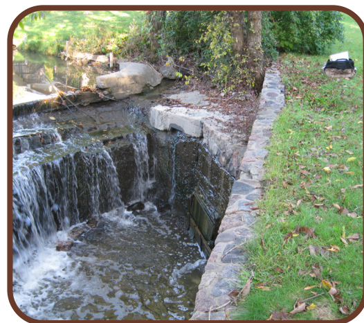
Danvers Pond dam prior to restoration
