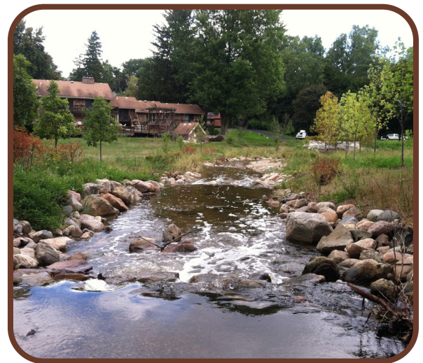
Stream restoration complete
